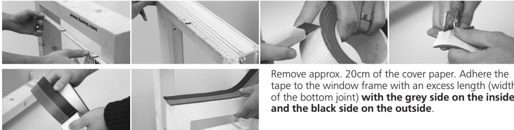
Remove approx. 20cm of the cover paper. Adhere the tape to the window frame with an excess length (width of the bottom joint) **with the grey side on the inside and the black side on the outside**.
